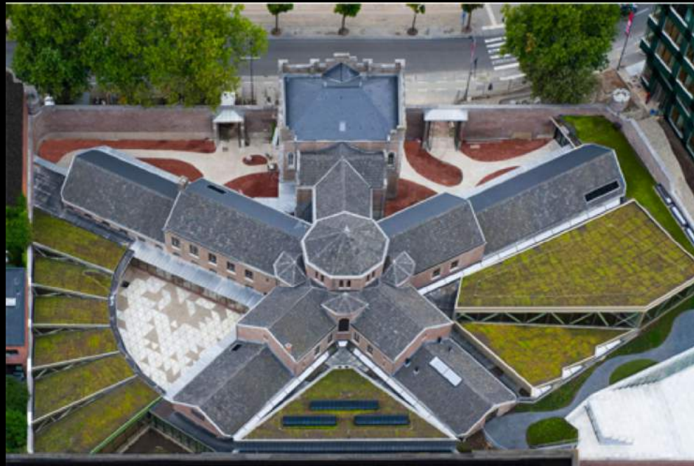
The 19 th century Prison of Hasselt as an adaptive reuse project for the Faculty of Architecture & Arts / U Hasselt
