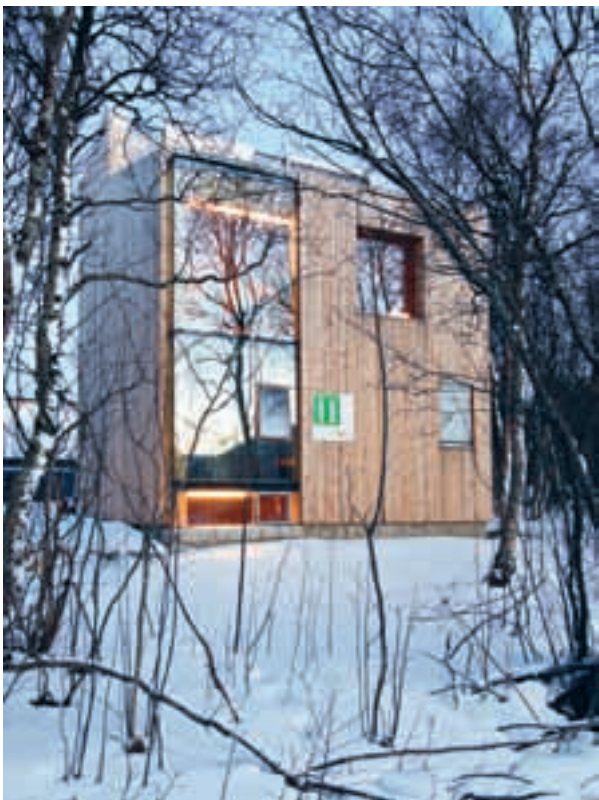
[1.2] I-BOX, Norway's first passive house, Tromsø (Steinsvik Architects Office AS)
