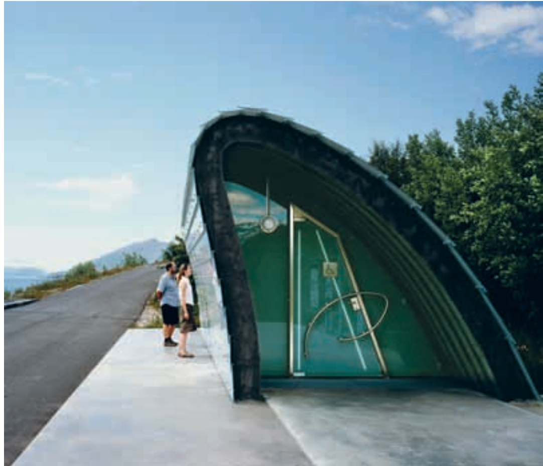
[5.5] Toilet and services building at Hellåga rest area on the Coastal Realm Highway near Sjøna in Rana. National Tourist Route, Helgeland North (Nordplan AS - Arild Waage)
