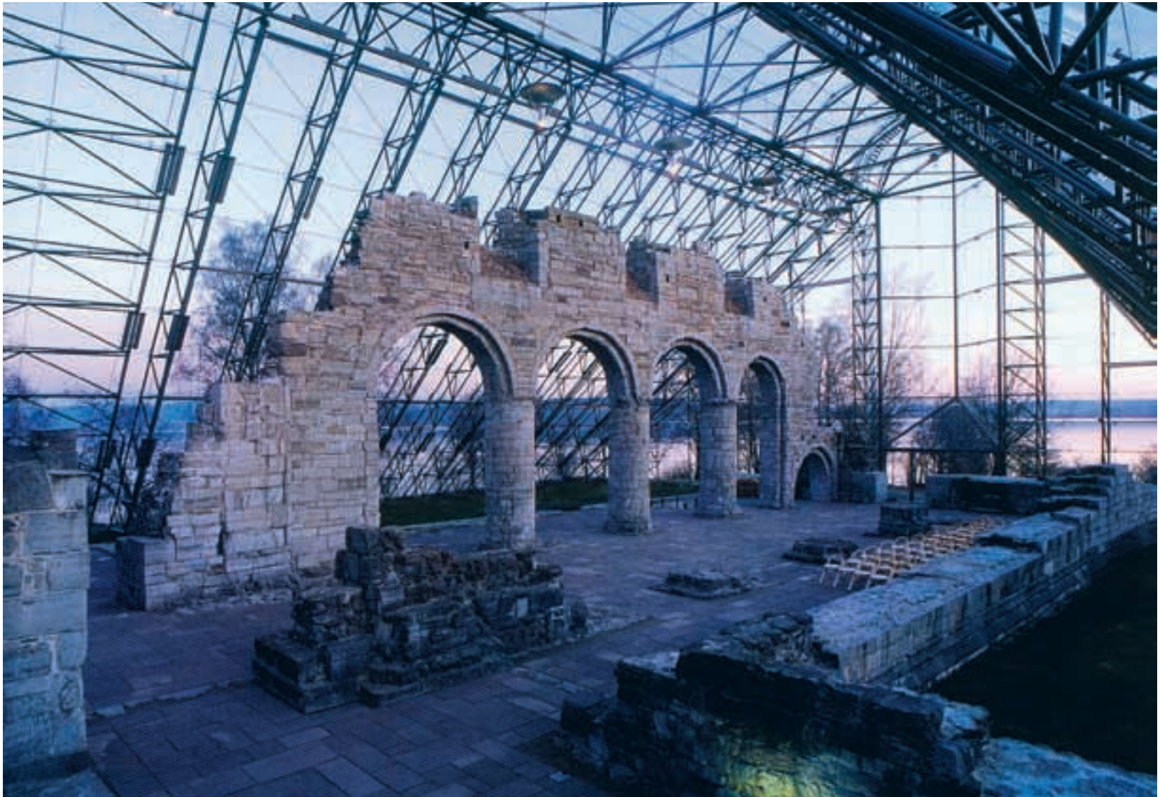
[3.4] Cathedral Headland, Hamar (Lund + Slaatto Architects AS)
