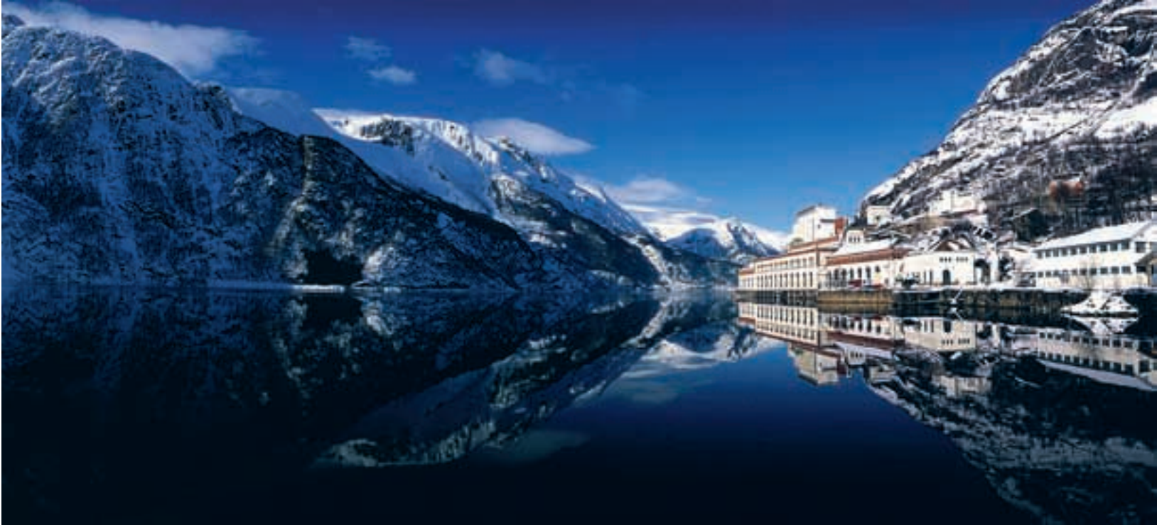
[2.7] Tyssedal power station. Odda, Hordaland.
