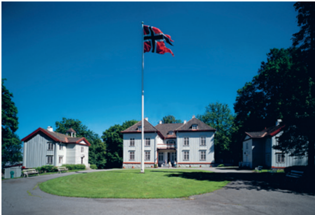
[3.6] The Eidsvoll building of 1770, Eidsvoll.
