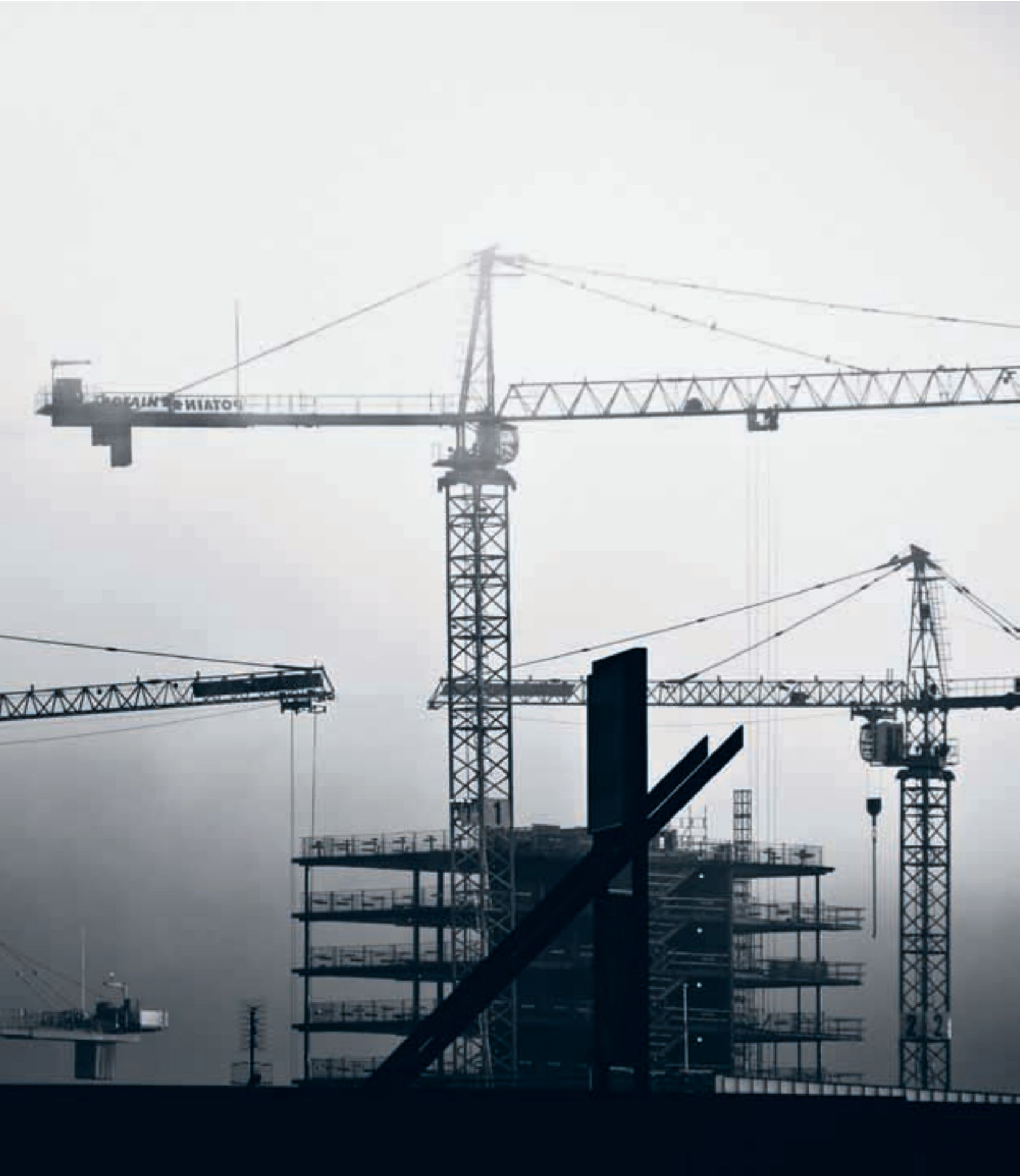
[0.7] Building site. Bjørvika, Oslo
