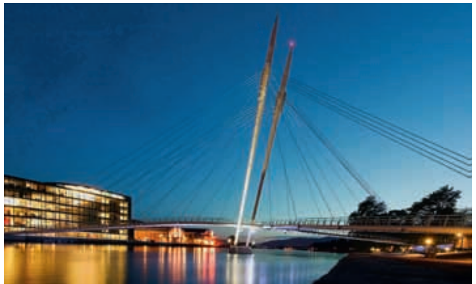
[6.2] Winner of European Steel Bridge Award 2008: Ypsilon pedestrian and cycle bridge. Drammen (Arne Eggen Arkitekter AS)
