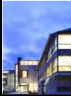
Page: 30 Food Safety Office, Backweston Co. Kildare Architect: OPW Architectural Services Client: Department of Agriculture, Fisheries and Food Photo: Gerry O'Leary
