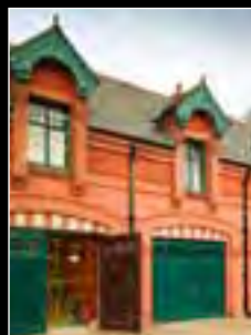
Page: 46 The Red Stables, St. Anne's Park, Mount Prospect Avenue, Dublin 3 Architect: Dublin City Council Client: Department of Culture, Recreation and Amenity, Dublin City Council Photo: Ros Kavanagh
