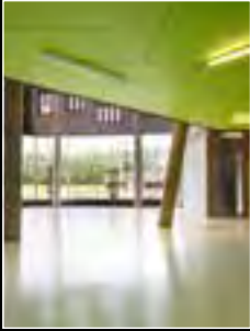
Page: 58 Ratoath College, Co. Meath Architect: McGarry Ní Éanaigh Architects Client: County Meath Vocational Education Committee Photo: Richard Hatch Photography
