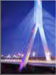
Page: 52 Boyne Bridge, M1 Northern Motorway Engineer: Roughan & O'Donovan Client: Meath County Council and Louth County Council Photo: Ros Kavanagh
