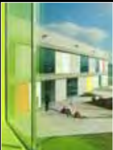
Page: 54 Brookfield Community Youth Centre and Crèche, Tallaght, Dublin 24 Architect: Hassett Ducatez Architects Client: South Dublin County Council Photo: Michael Duffy
