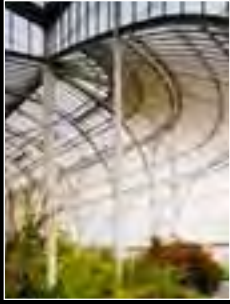
Page: 26 National Botanic Gardens of Ireland, Glasnevin, Dublin 7 Architect: OPW Architectural Services Client: The Commissioners of Public Works Photo: Ros Kavanagh
