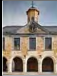
Page: 20 The Main Guard, Sarsfield Street, Clonmel, Co. Tipperary Architect: Margaret Quinlan / OPW Architectural Services - National Monuments Client: The Commissioners of Public Works Photo: Ros Kavanagh
