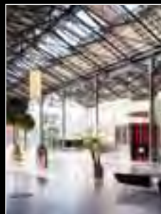
Page: 45 former Stack A Tobacco Warehouse, now The CHQ Building, Custom House Quay, Dublin 1 Architect: Michael Collins Associates Client: Dublin Docklands Development Authority Photo: Ros Kavanagh
