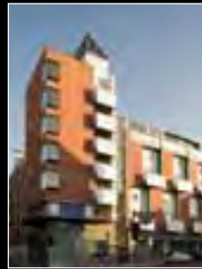
Page: 22 York Street Housing, York Street, Dublin 2 Architect: Seán Harrington Architects Client: Dublin City Council Housing and Residential Services / City Architects Department Photo: Seán Harrington Architects and Philip Lauterbach
